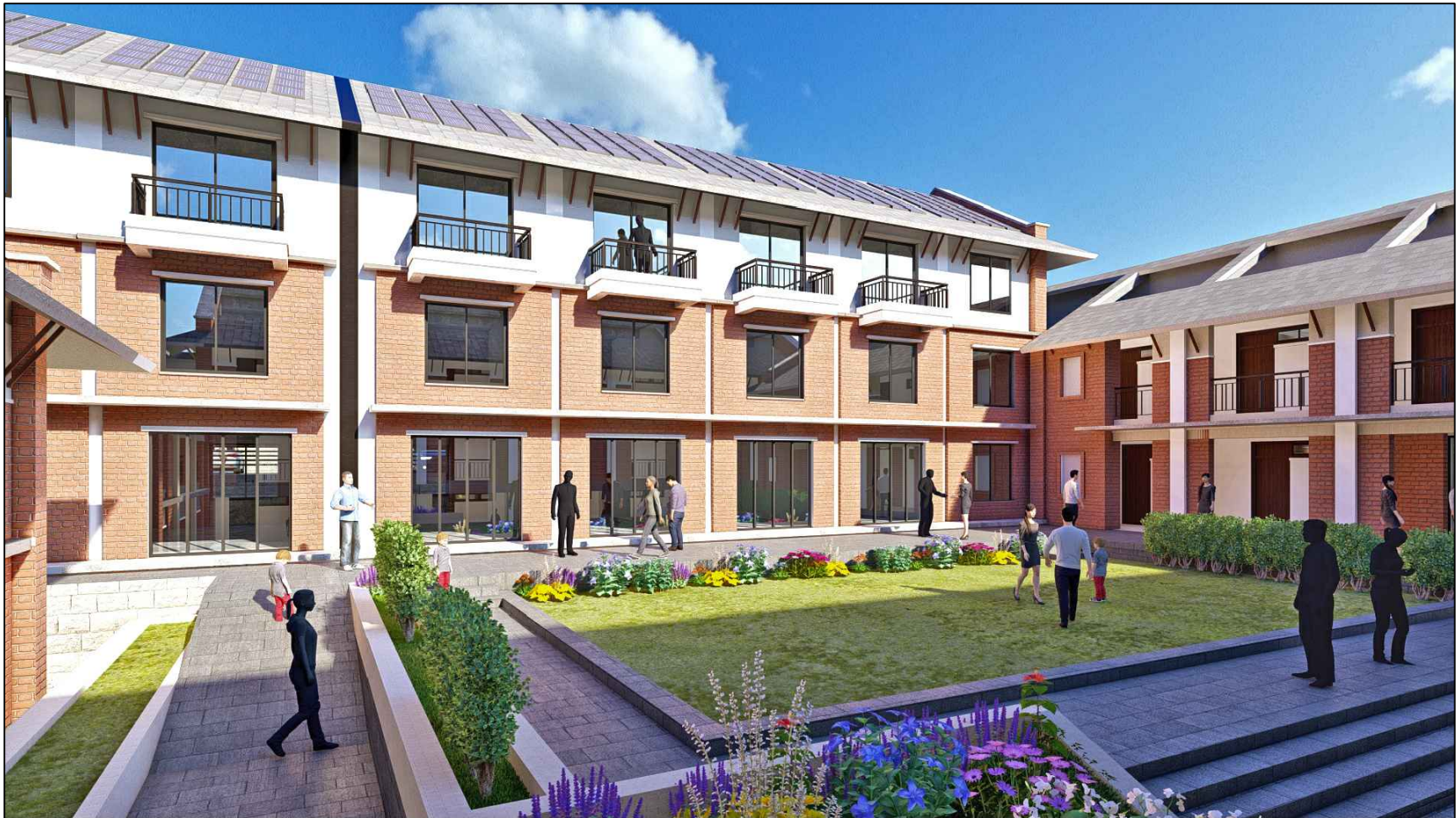
VIEW OF THE COURTYARD FROM THE SOUTH BLOCK
