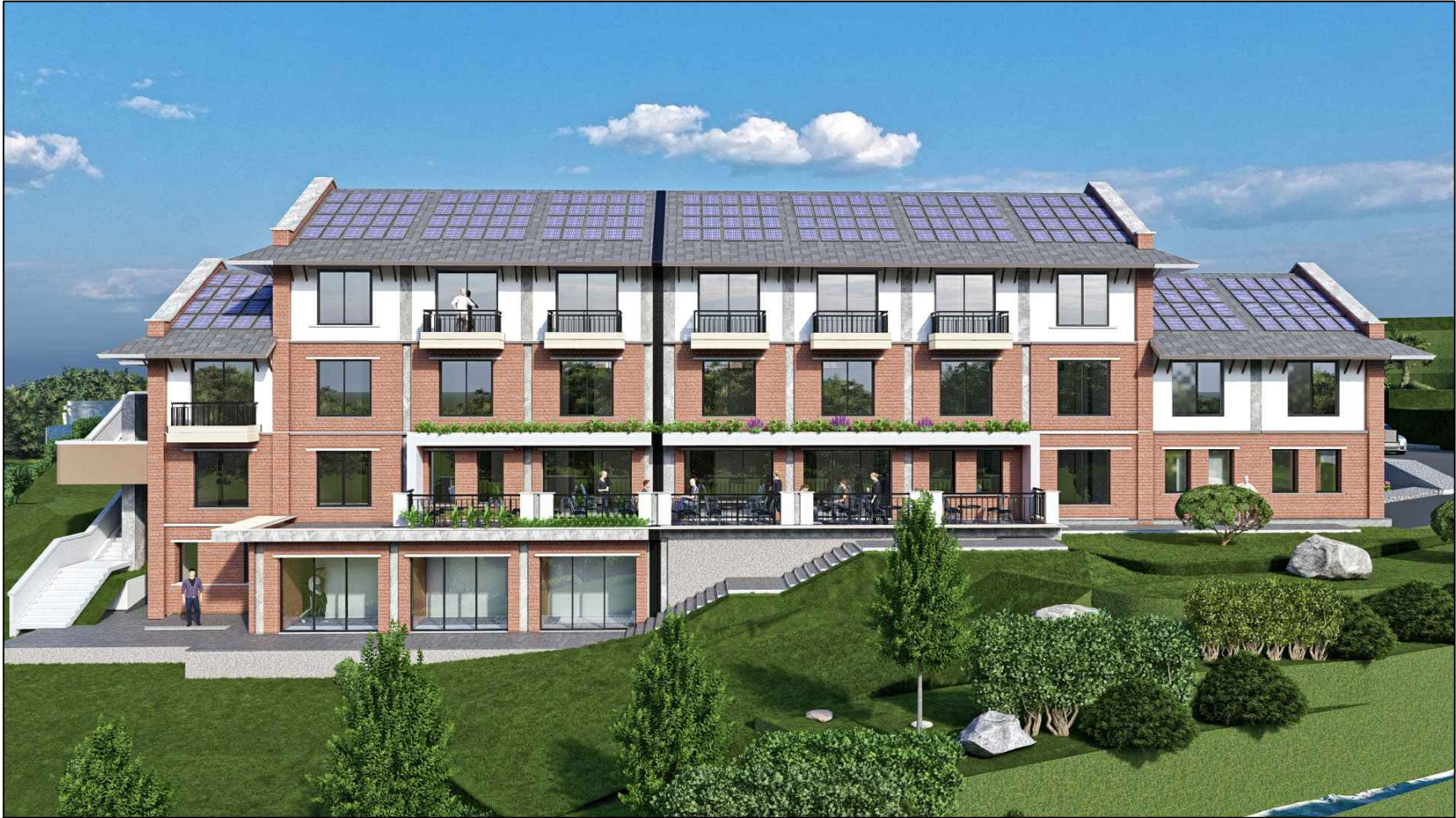
SOUTH ELEVATION OF THE BUILDING
