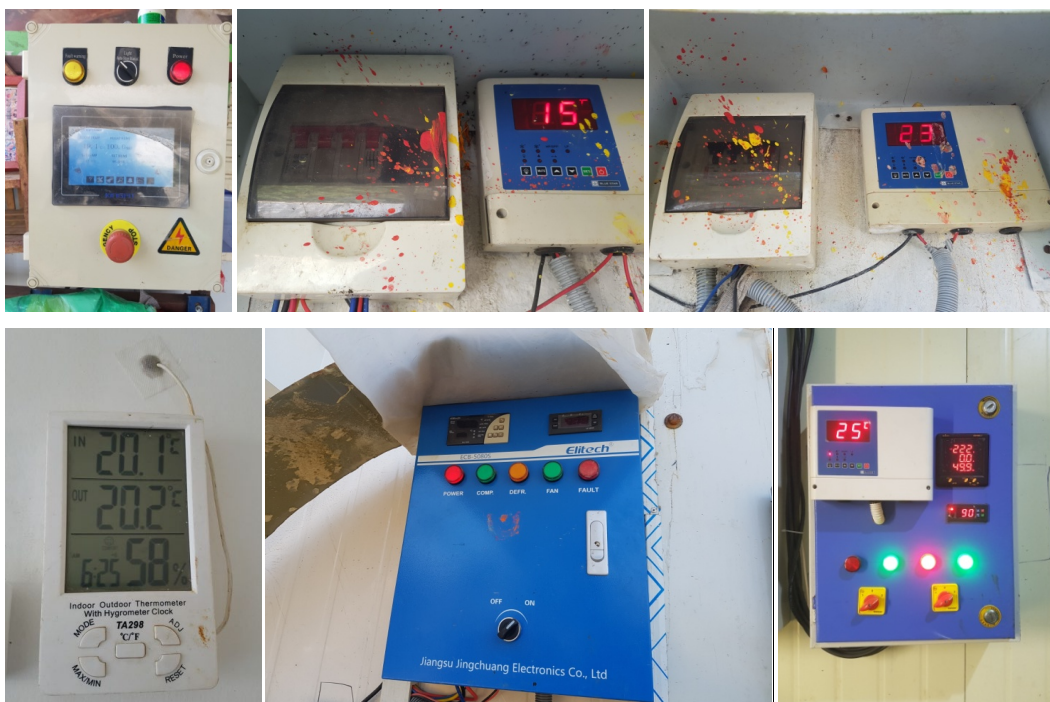
Fig. 14. Control panels showing temperature, humidity, CO 2 concentration etc outside of the incubation rooms.
