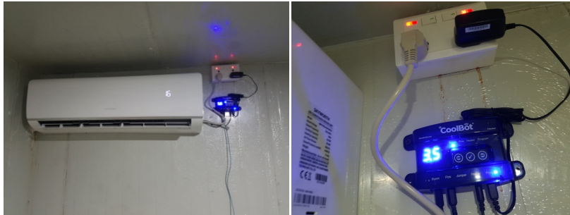
Fig. 10. Application of CoolBot technology for lowering temperature of cold storage up to 4C or lower.
